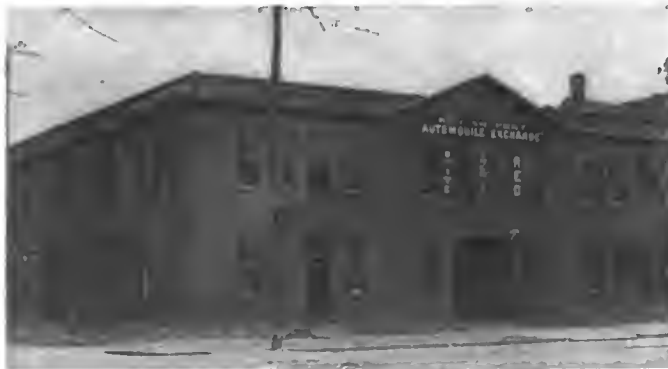
GARAGE OF THE WILLIAMSPORT (PA.) AUTOMOBILE EXCHANGE.
